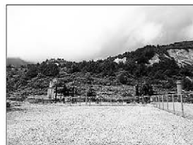
Fig.6 : production wells in production station
