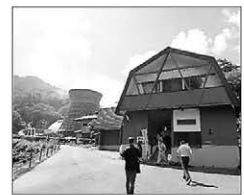
Fig.1 : Matsukawa Geothermal Museum and a huge cooling tower
